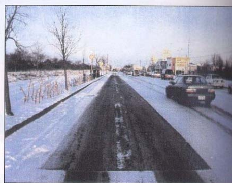
Fig. 21.14 The GPUX surface applied in a winter climate, Hokkaido, Japan. The dark areas are ice-free strips of GPUX material (the elastic compression/expansion under the rolling tyres break up and remove any ice). From [Potter, 1996], used with permission.
