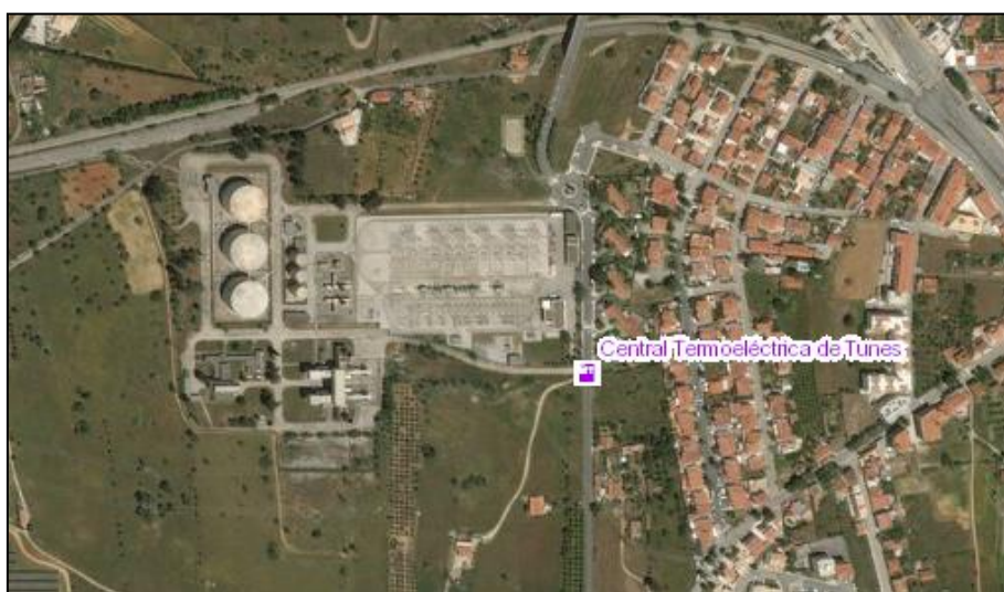
Figura 78 – Central Termoelectrica de Tunes
