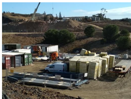
B – Lã mineral a instalar na nave industrial
