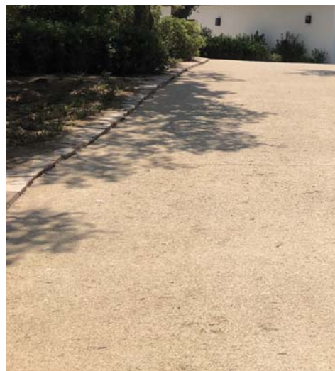
Two main roads that will allow buggies to circulate between the different main spots of the resort will be made of stained the mass concrete. Aggregates from the site will be cast in the cement to confer it a very rustic look. These roads will stick to the ancient roads shape that are already flattened and immobilised grounds (see bellow).
