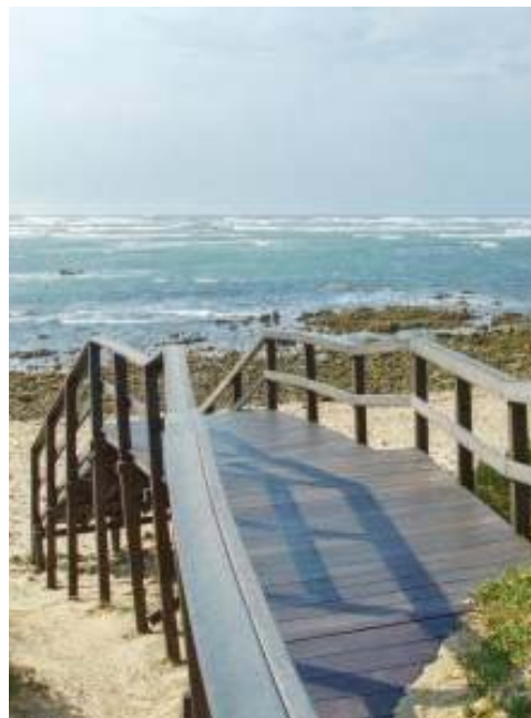
Two different types of wooden walkways are proposed. Elevated path will preserve the dunes and avoid erosion due to pedestrians.
